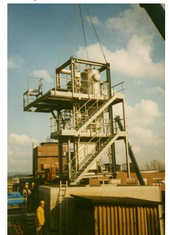
...and preassembled in a steel frame
